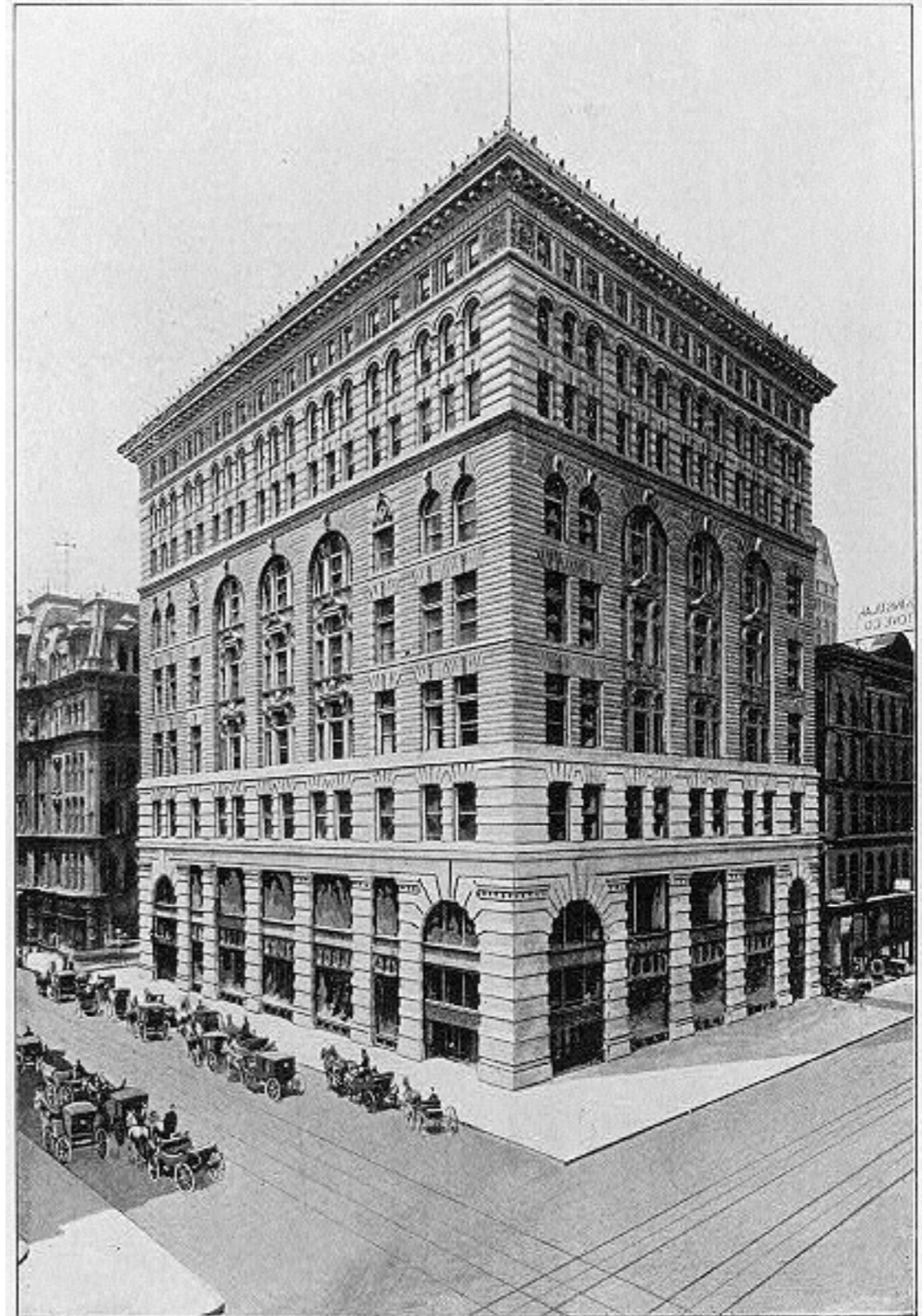
MARSHALL FIELD'S BUILDING, ANNEX TO RETAIL STORE, WABASH AVENUE AND WASHINGTON STREET.
